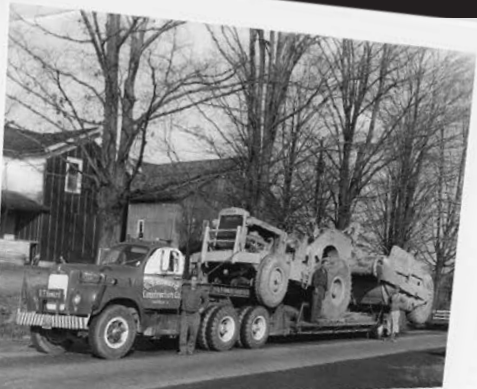
G. F. Howard Construction of Carroll, Ohio, has brought this Cat 950D from New York, New York. Note that the rear axle is suspended off the back of the body. (Courtesy of Larry Kohlman, HCEA Archives)
